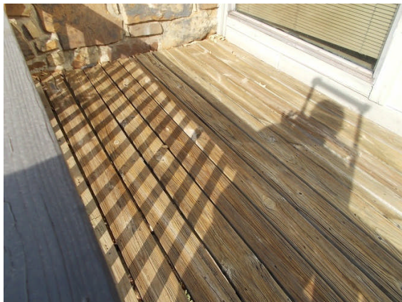
24. 2x6 treated decking.
