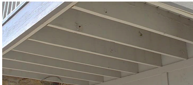
8. Joists appear normal. 2x10@16; cantilevered.
