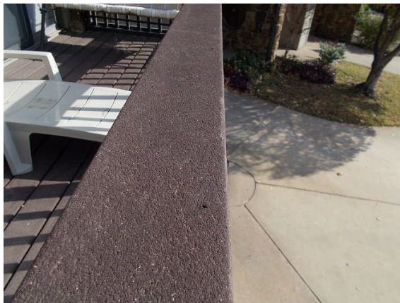
12. Synthetic Trex material used for handrail cap also. Nice.
